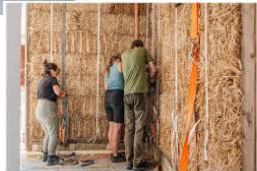
Formation sur chantier rebuiLT, Eoullens 2023 © rebuiLT, EPFL
